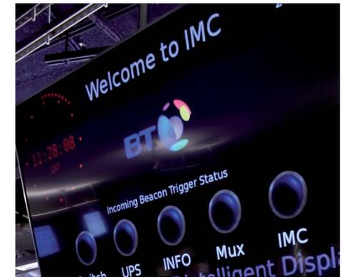
VSC. The IMC was designed to last well into the future with 39 operational monitoring positions, each with multiple screens and tablets, combined with traditional rack mount panels close by. Besides these, monitor walls display a mix of baseband and PC-originated signals.
